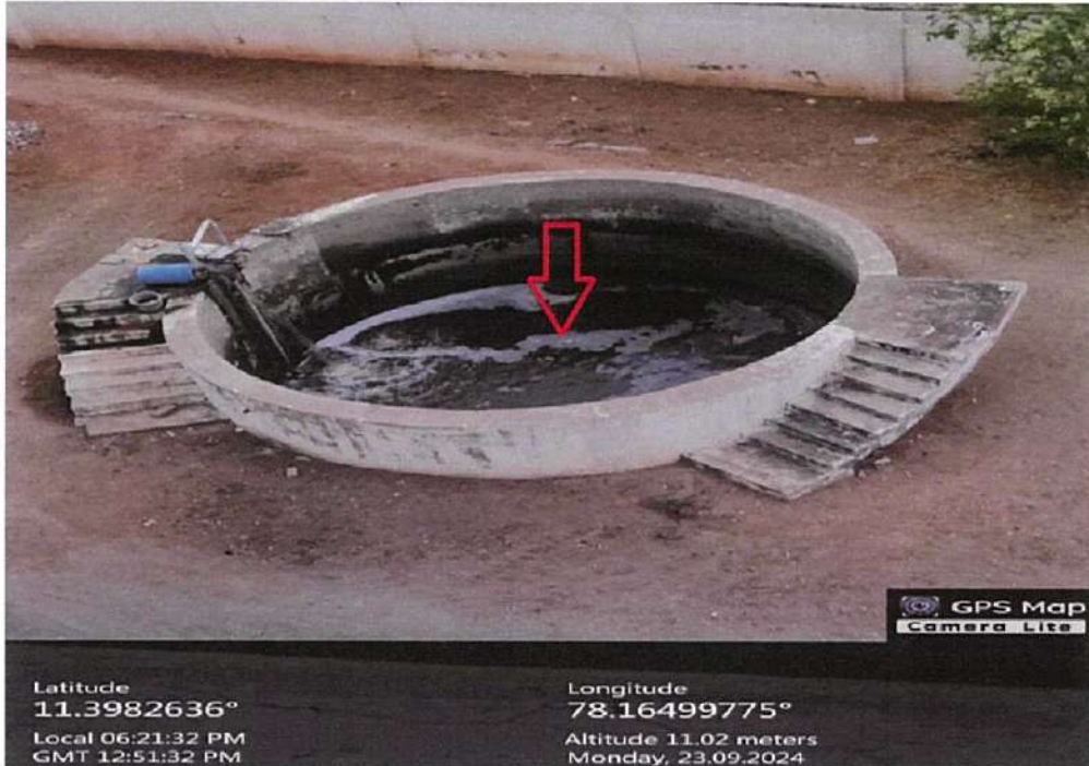
Wastewater storage well
