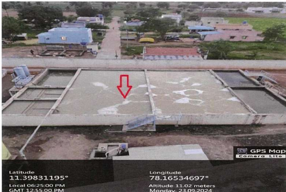
Wastewater Recycling Plant
