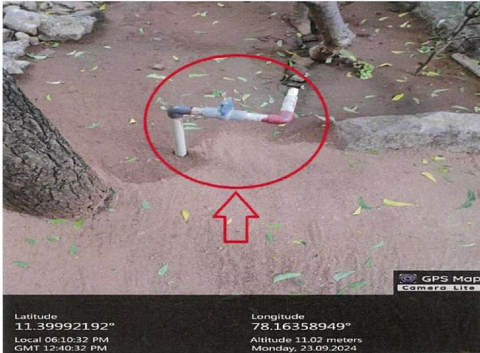
Recycled Water Supply to the trees
